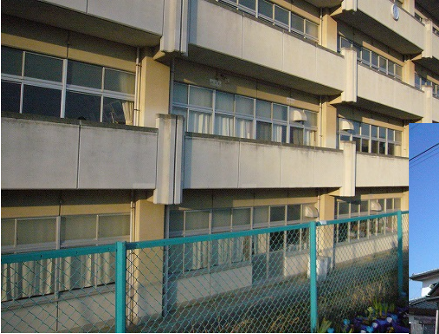
Virtually no severe damage around IBR003, 1.6g site.
