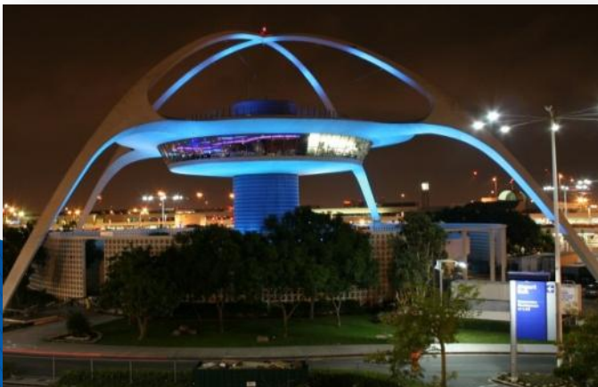
Testing Retrofit of LAX Theme Building
