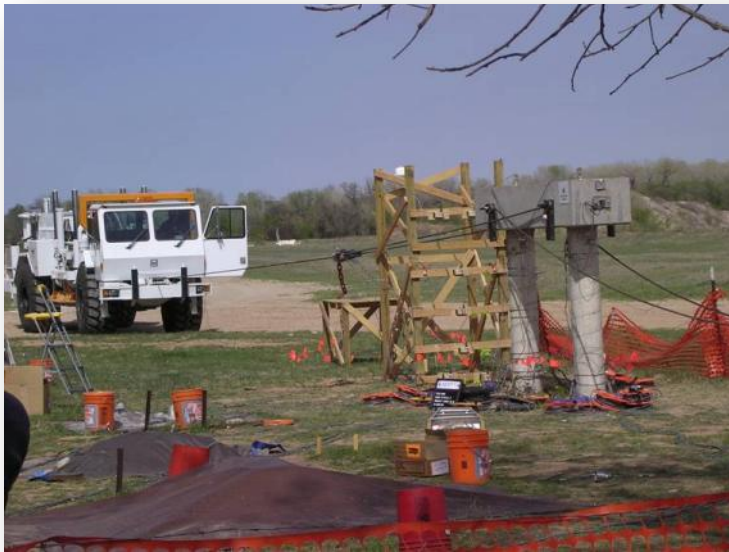
1/4 scale bridge bent
