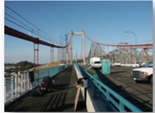
Monitoring Carquinez Bridge
