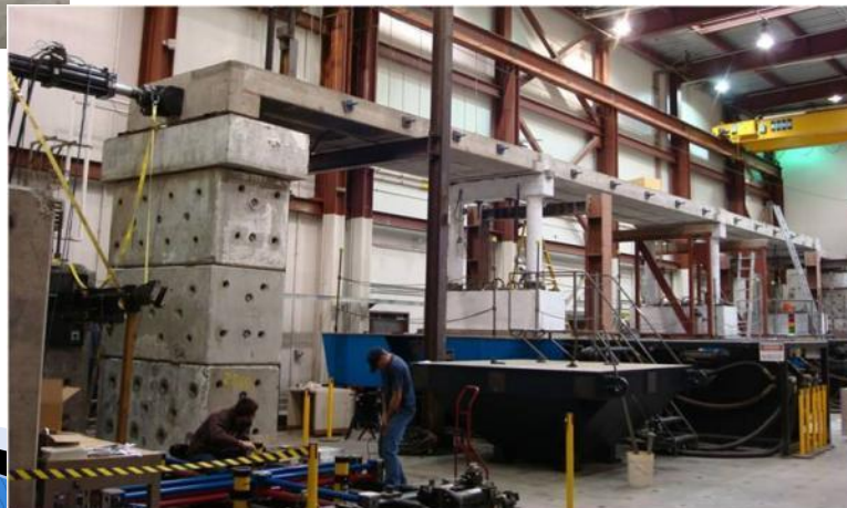
110-ft-long, 200-ton, 4- span bridge
