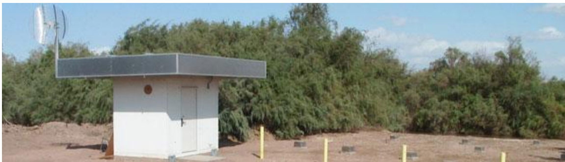
Fig. 2. The NEES WLA facility just after construction was completed in 2004
