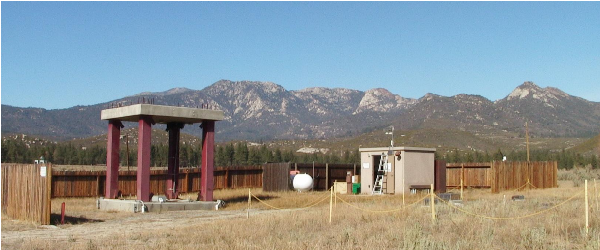
Fig. 1. Panoramic View of the NEES Garner Valley Facility in 2008.
